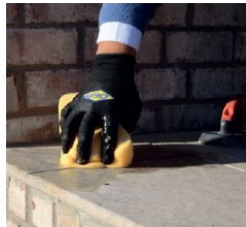
PIC 2. Remove excess grout with clean water.
