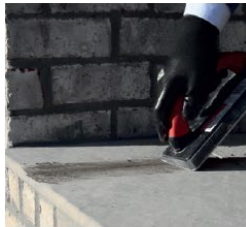
PIC 1. Fill joint with grout.
