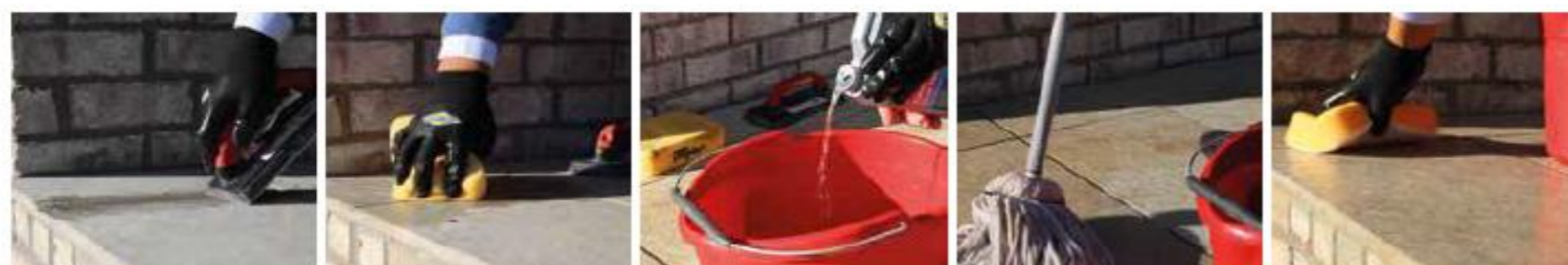
PIC 1. Fill joint with grout.
