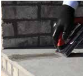
PIC 1. Fill joint with grout.
